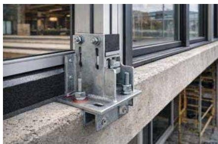
Masonry support and facade elements
