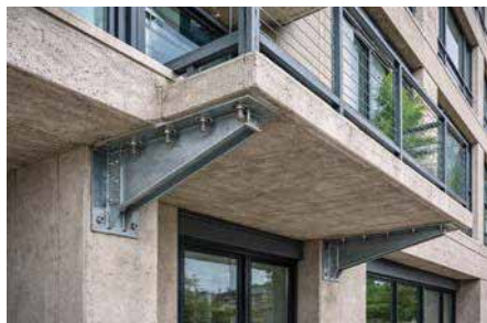
Balcony parapets and canopies
