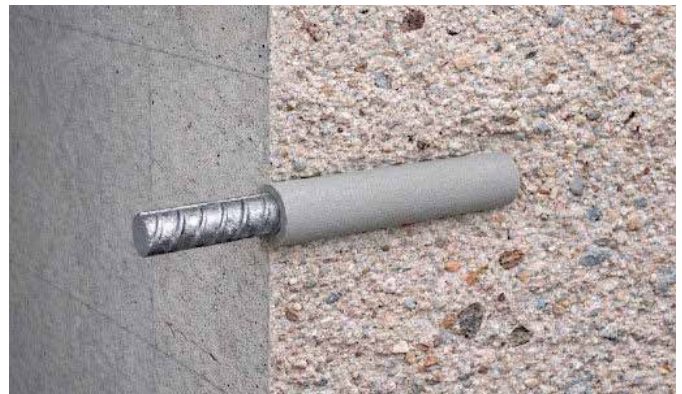
Rebar anchored to concrete
