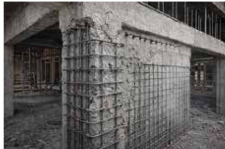
Reinforcement of structures
