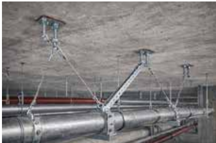
Seismic bracing
